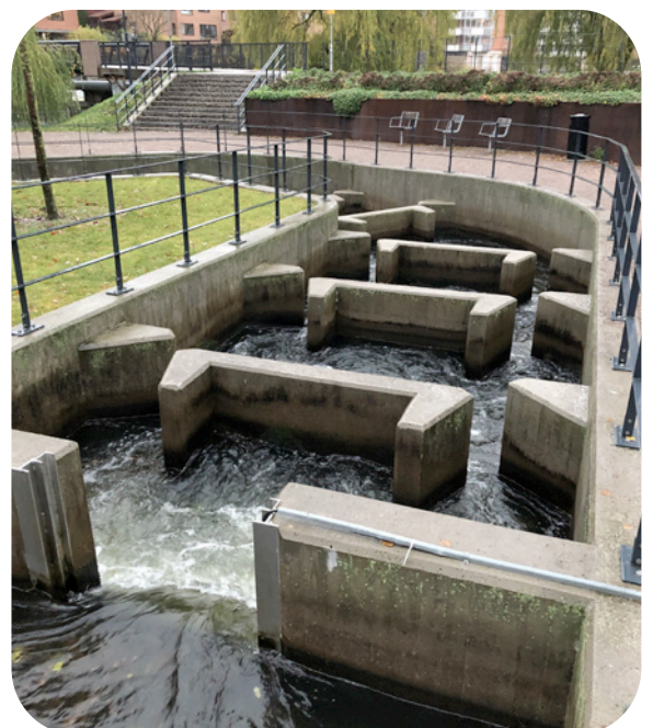
Photo 3. Fish ladder made of concrete, 2019, Sweden © Johan Kling.
