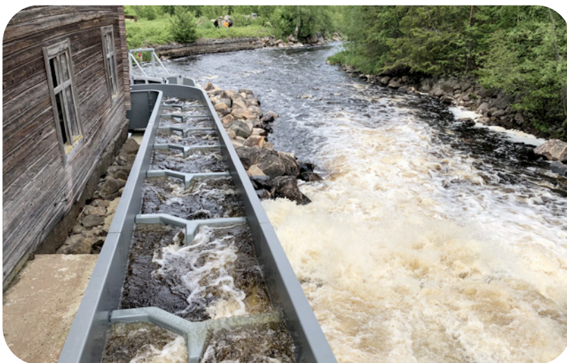
Photo 2. Fish ladder made of composite, 2019, Sweden © Johan Kling.
